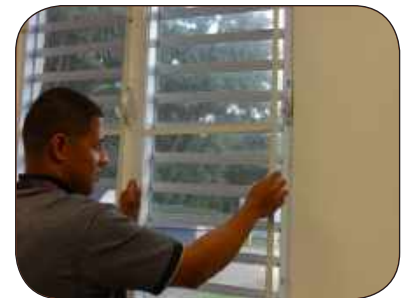
Install or repair window & door screens.
